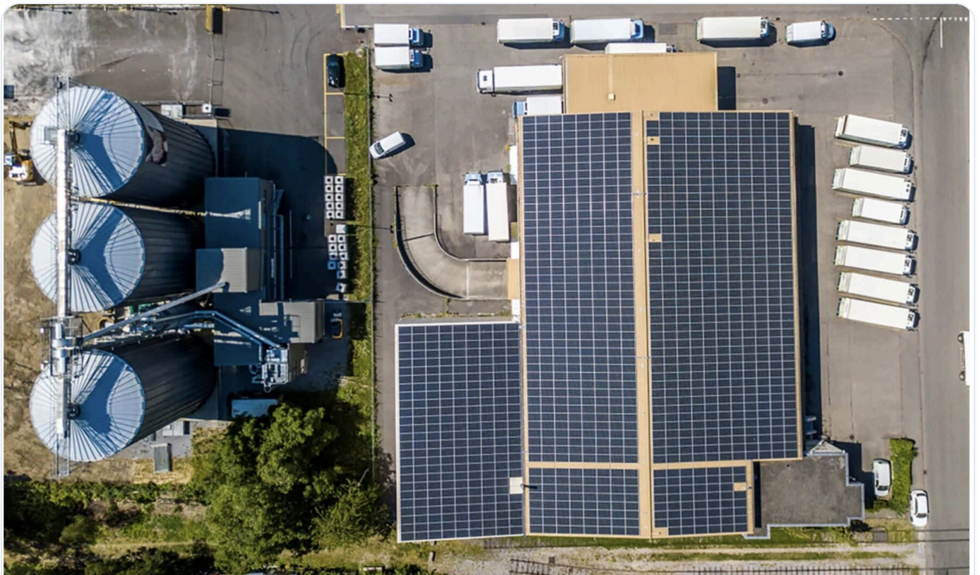
Installation agrocommerciale (grain / meunerie)
