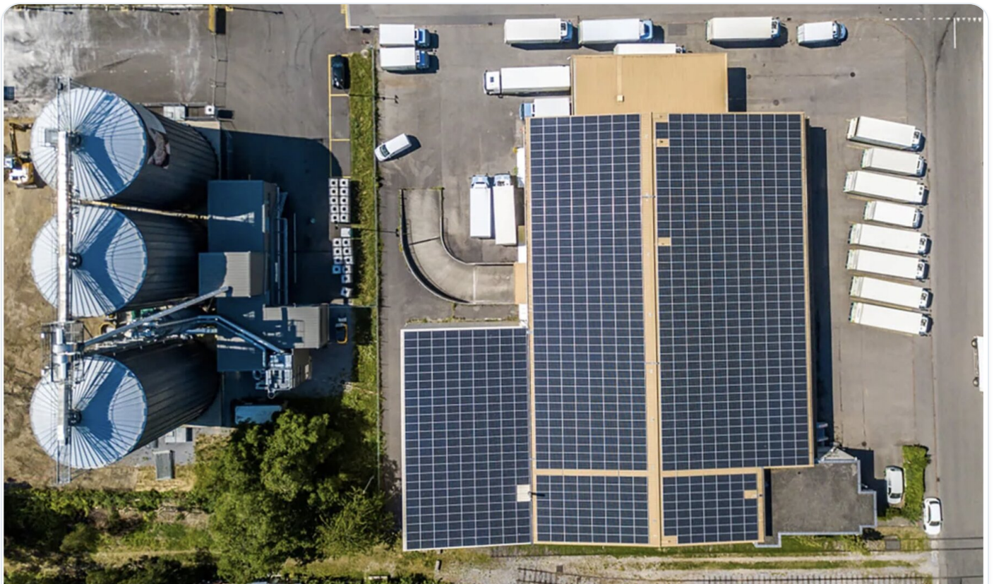
Installation agrocommerciale (grain / meunerie)
